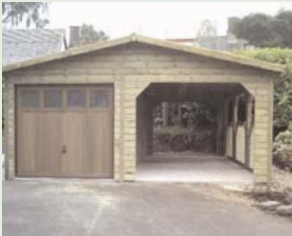
Garage and carport with up and over cedarwood door
